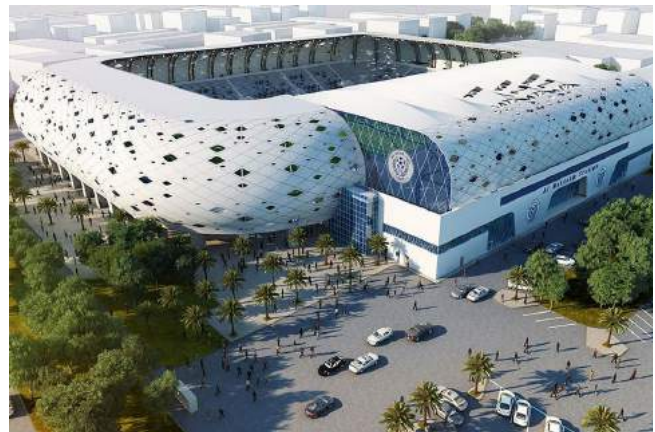
Al Maktoum Stadium, Dubai
