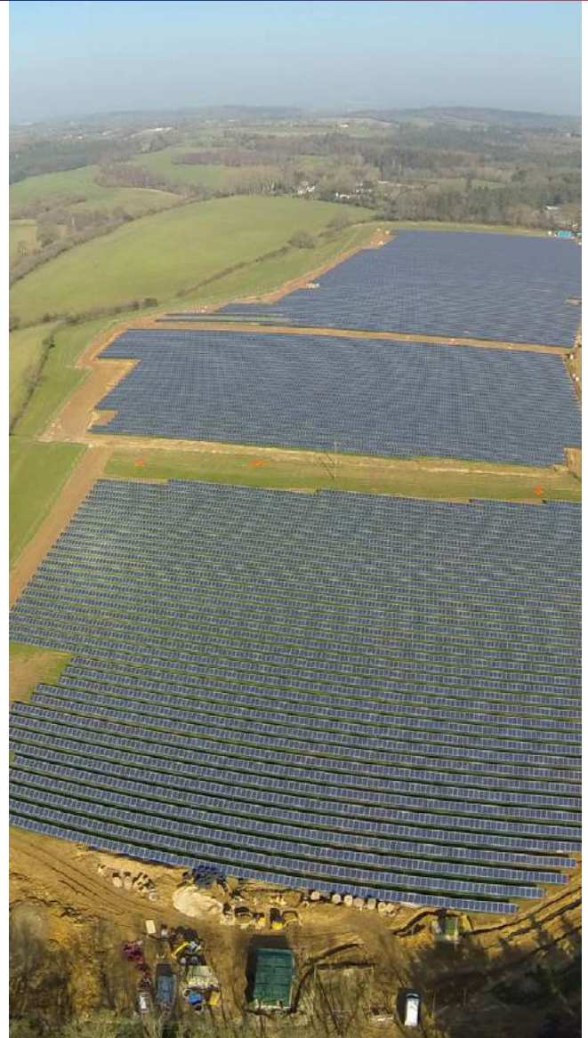
Solar farm constructed in Dorset, UK totalling near 7MW and 26,923 solar panels
