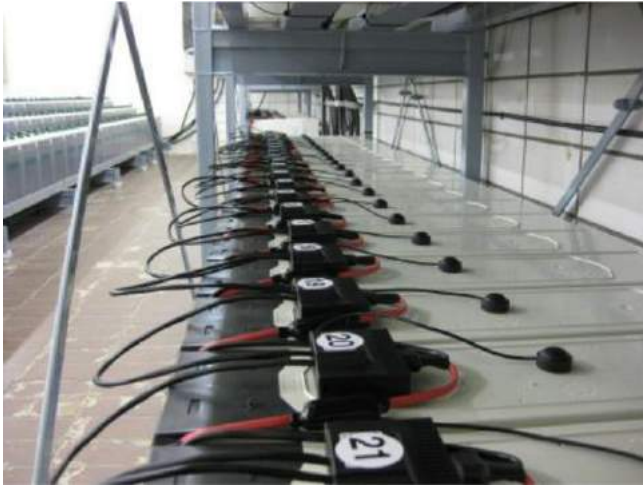
Civil Aviation Authority Installation, Europe
